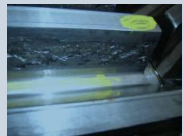
Typical condition of the tooth flanks in September 2006 Sharp edged pitting on tooth flanks
