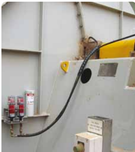
perma STAR VARIO remote mounted to a fan jack shaft providing safe access for inspections and servicing.
