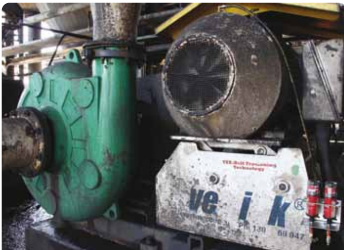
Application Motor driving Krebs slurry pump Lubricator STAR VARIO L250 Install Kit K230C
