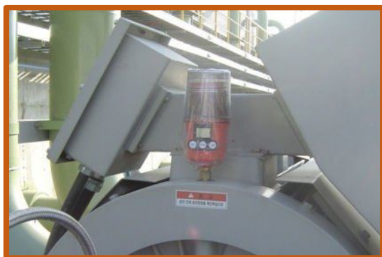
Fan bearing – direct mount 250cc Pulsarlube (Order Code 91-GL250)
