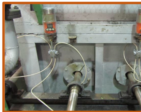
Fan bearing – 4 outlet divider valve 250cc Pulsarlube Customer supply tube and fittings (Order Codes 91-GL250 & 41-LBK-4-000-O-BRA)
