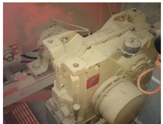
Bearing and seal grease lines
