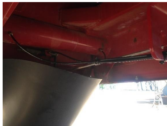
Suspension grease lines
