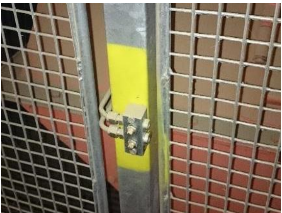
2 outlet grease anchor block
